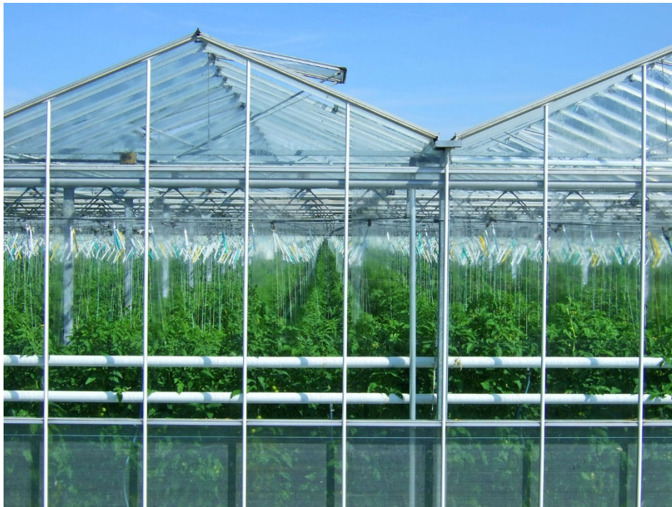
Figure 3.3 Typical Venlo type greenhouse
